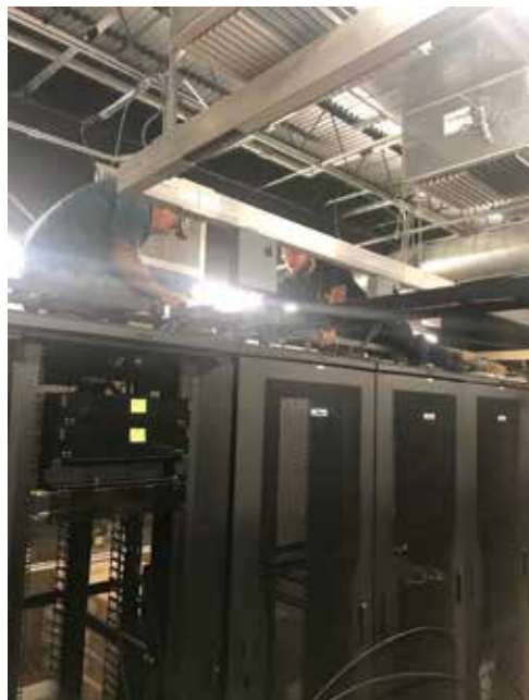
Fiber Optic Cable Installation
