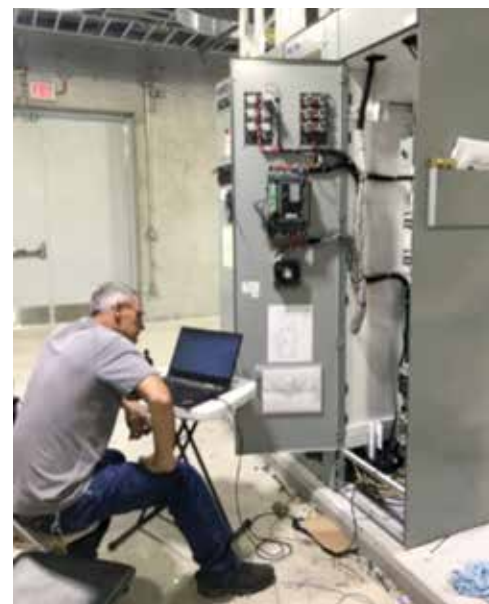
Paul Hardin, SCADA Technician works diligently at the East Canal Pump Station to install and setup VFD's for improved and remote operations of the pumps and motors.
