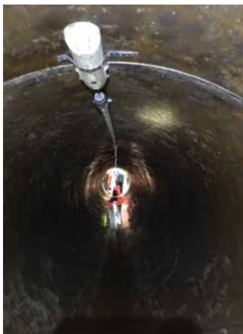
As part of SCADA implementation, Highlands Division and SCADA staff installed an in-pipe flow meter in the 48-inch pipe located at SJRA's HCFCD Siphon structure in Baytown.
