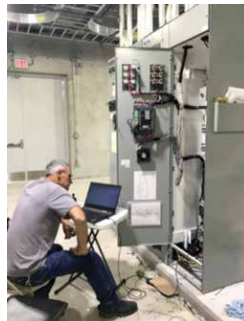
Paul Hardin, SCADA Technician works diligently at the East Canal Pump Station to install and setup VFD's for improved and remote operations of the pumps and motors.
