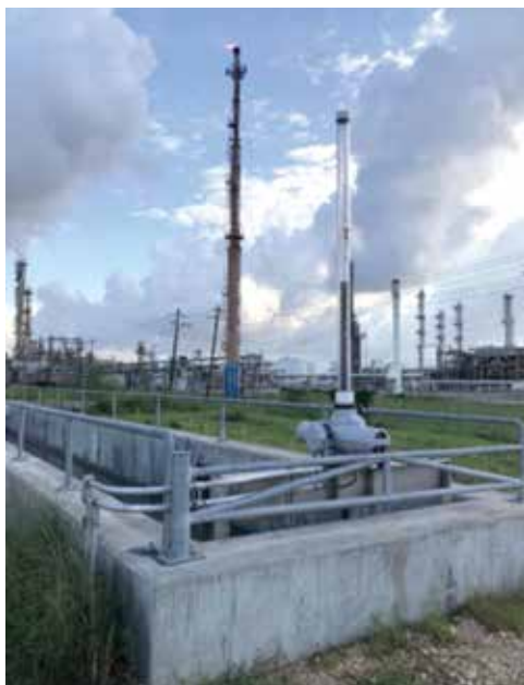
Actuators installed on gate control structures located adjacent to industrial customers provide for improved and remote operations.
