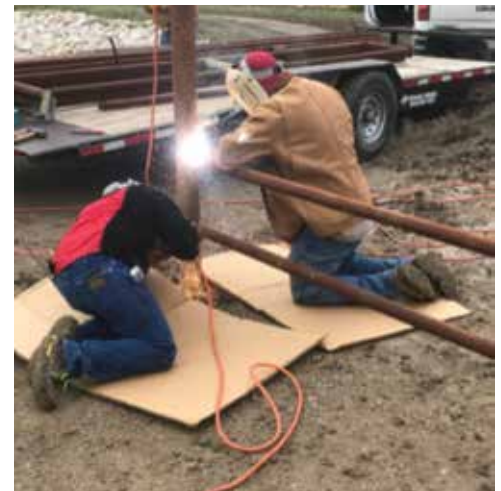
Division staff, Bryan Kilgore and Jay Jones assist in the effort to improve access and security through the placement of pipe gates and fencing at the Wallisville Road Siphon structure.
