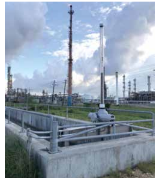
Actuators installed on gate control structures located adjacent to industrial customers provide for improved and remote operations.
