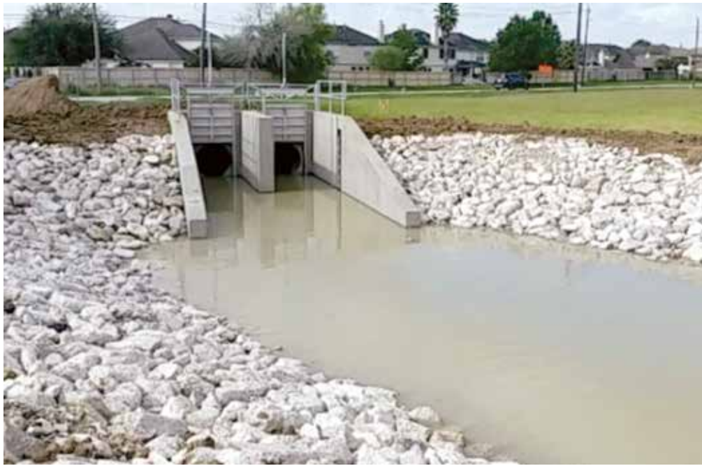
Wallisville Road Siphon structure (two 48-inch pipe) is the most recent siphon project completed on the East Canal. The new structure provides for redundancy and improved reliability. Coordination and cost sharing occurred between SJRA and Harris County on this structure.
